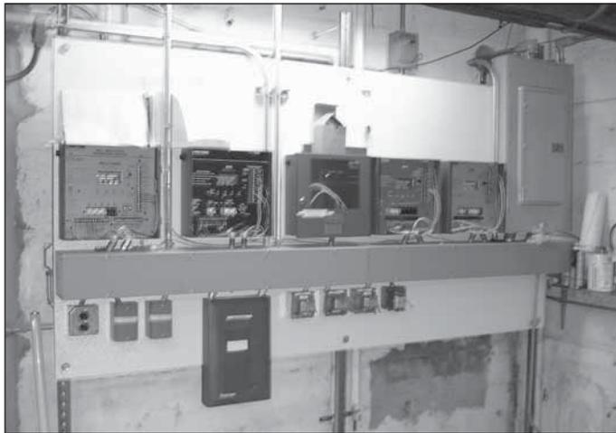
*Each Heat-Timer control provides unique adjustment capability to maximize the efficiency of each individual system. Remote communications allows for local and/or remote adjustments.*
