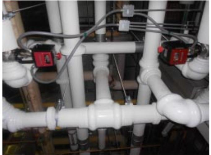
*Two 2-inch Heat-Timer ETV stainless steel valves installed in parallel in the Hilton’s domestic hot water piping.*
