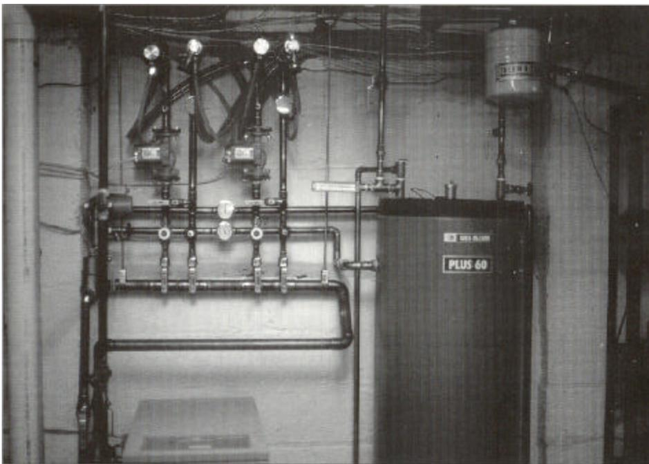
*The InjecTemp injects hot water from the boiler loop into the radiation loop as needed to maintain comfortable indoor temperatures.*
