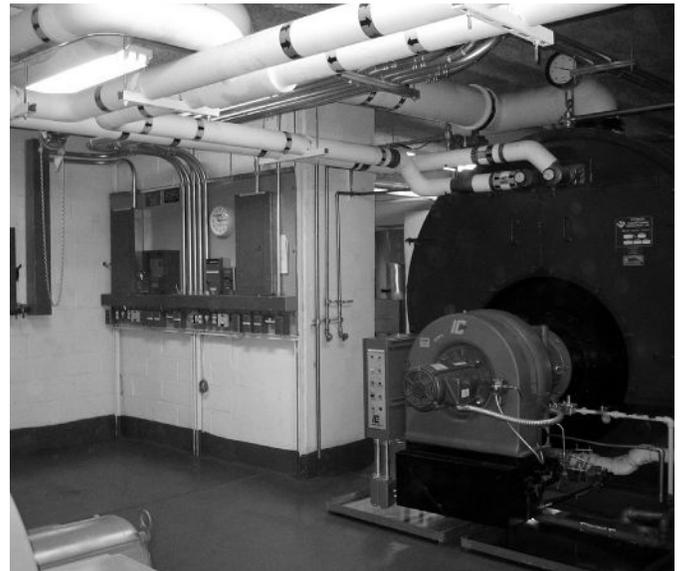
*Heat-Timer Multi-Mod controls provide modulating control of the two new Scotch Marine type, 3-pass boilers installed at Kips Bay.*
