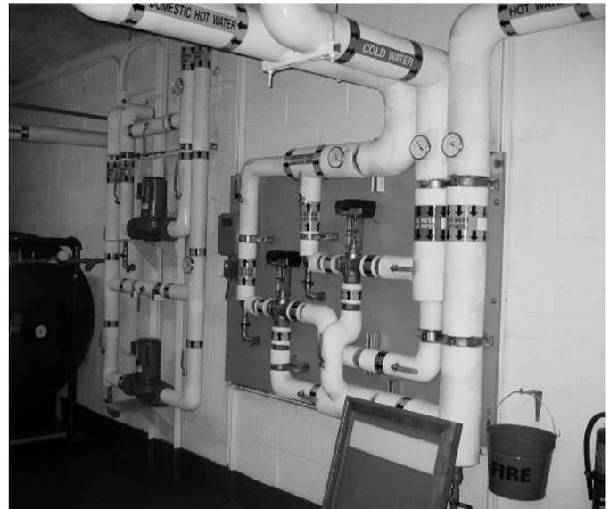
*Heat-Timer ETVs (Electronic Tempering Valves) mix hot and cold water accurately to provide a safe domestic hot water temperature of 135°F at Kips Bay.*
