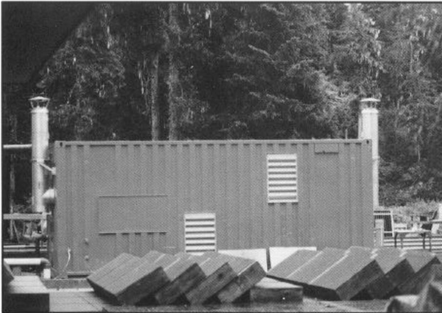
*Because the hatcheries were so remote (3 of the 4 were accessible only by boat or plane) the units had to be built elsewhere and then transported to the site. Therefore they had to be mobile, and containerized for protection against the elements.*
