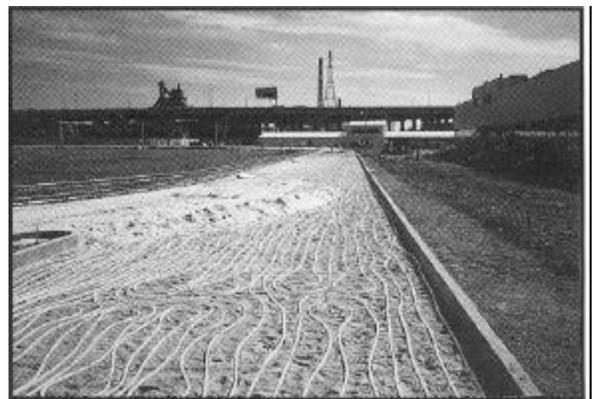
*Over 6 miles of radiant pex tubing was installed beneath the surface of the race track at Shoreline Star Entertainment Center in Bridgeport, CT*
