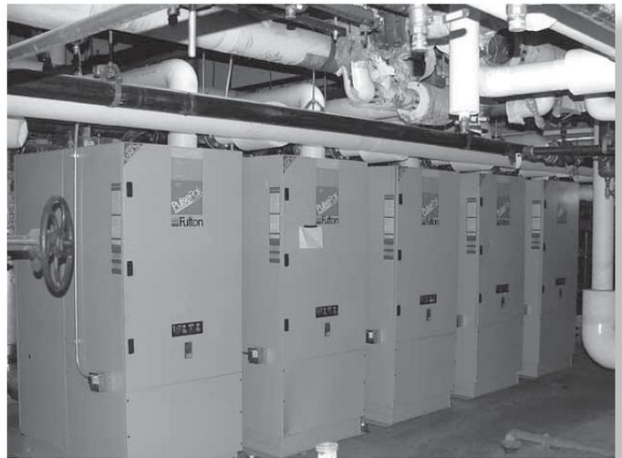
*A Heat-Timer Multi-Mod with an extension module provides modulating and lead lag control for five pulse boilers.*
