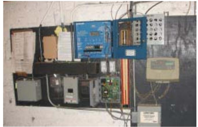
*116 Heat-Timer Platinum weather actuated controls were installed in Beach Lane Management properties.*
